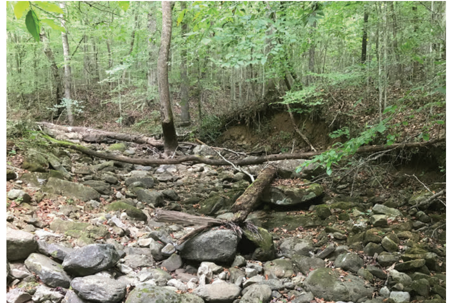
Downstream Conditions - Erosion at Barnes Branch & Lost Creek Confluence
