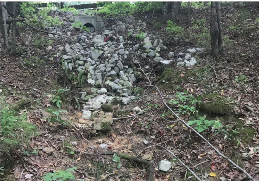
Existing Drainage System Outfall - Sewanee Elementary School
