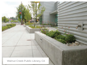
RAISED STORMWATER PLANTER
