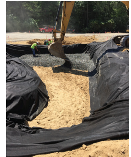
Confirming Elevations, Bottom of Bed Conditions, and Specified Fill Materials
