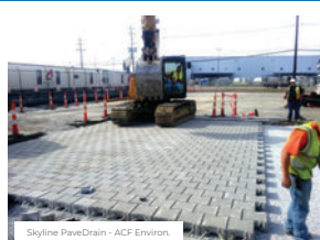
POROUS GRAVEL RESERVOIR
