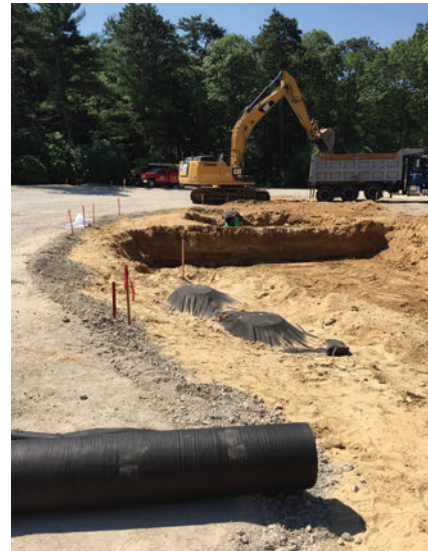
Confirming Elevations, Bottom of Bed Conditions, and Specified Fill Materials
