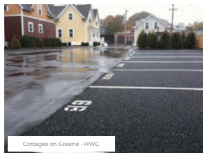
PERMEABLE PARKING STALLS
