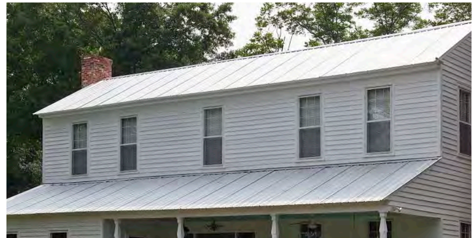
Below, a Folk Victorian house with a continuous eave with a shallow overhang.
