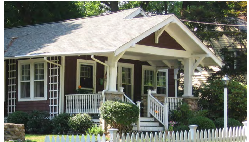
Above, the appropriate use of a nested gable for the porch of a Craftsman building. The nested portion of the roof covers the entire porch and shares the same roof plane on one side as the main roof.
