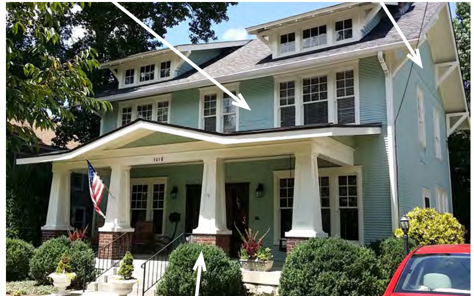
Both have deep porches with large, tapered wooden columns set on brick piers.
