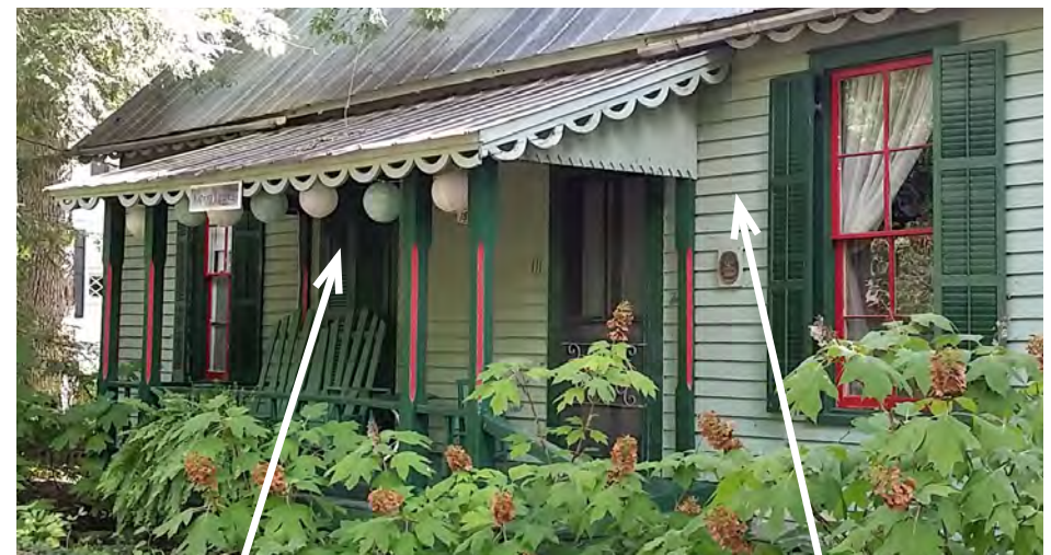
Simple shed-roofed porch with decorative scallop trim and two-color posts.
