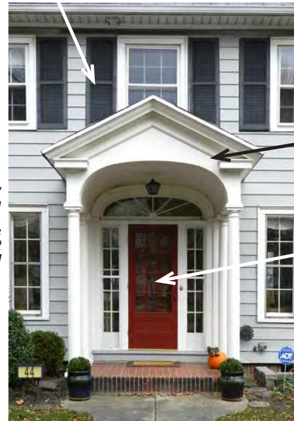
6-over-6 double-hung windows with appropriately sized shutters and trim.
