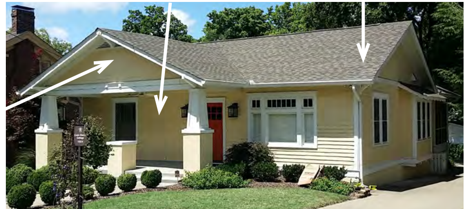
Low-pitched roof with deep overhangs.
