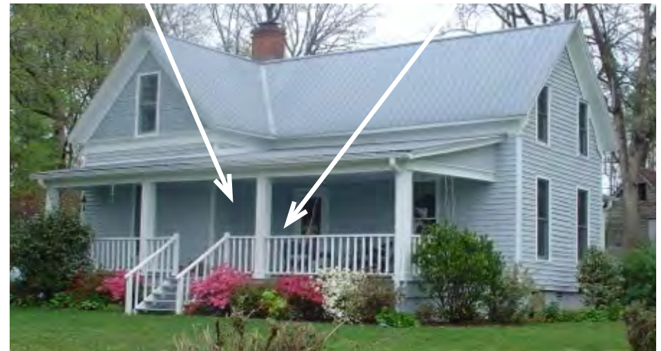
Simple square columns and railings on raised porch.
