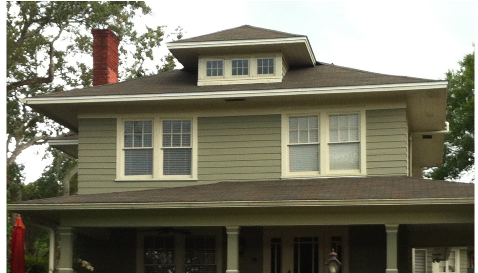
Above, a Craftsman house with a continuous, closed eave with a deep overhang.
