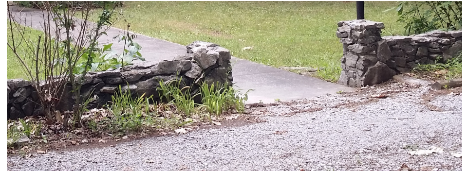
Stone Wall with Stone Piers
