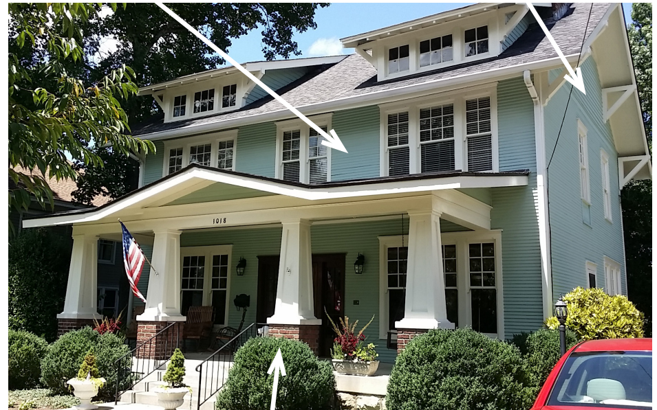
Both have deep porches with large, tapered wooden columns set on brick piers.
