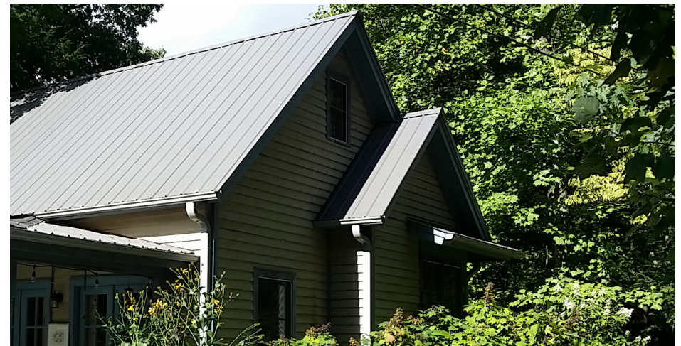
Below, the inappropriate use of a nested gable that is bumped out less than four feet, likely only to provide visual interest to the facade.
