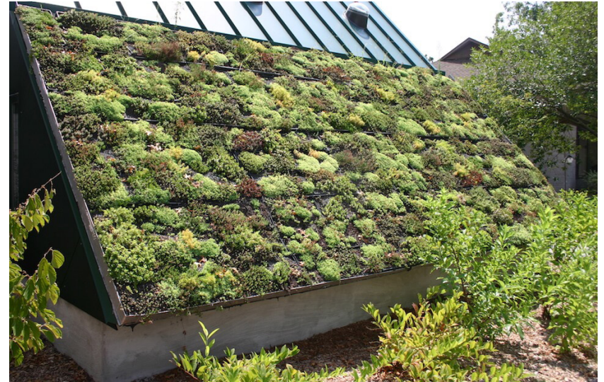
Green Roof Example
