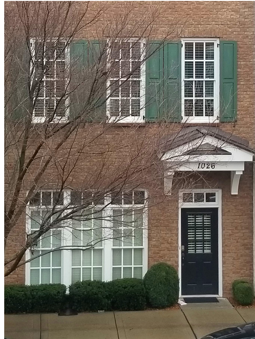
At right: Grouping of windows separated by mullions
